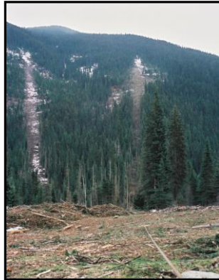
Figure 3. Harvesting narrow corridors with a cross-valley skyline system minimizes the need for roads.
